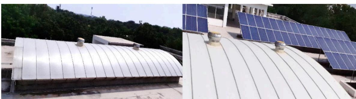
**Figure 9: Turbo ventilators**
