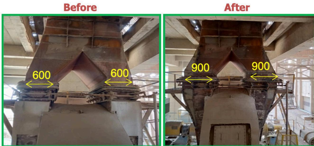
**As a result of the interventions, annual saving of INR 42 Lakhs from electrical energy savings (0.30 kWh / MT Clinker) and (0.1 kWh/MT Cement) was achieved in this fan inlet box modification.**
