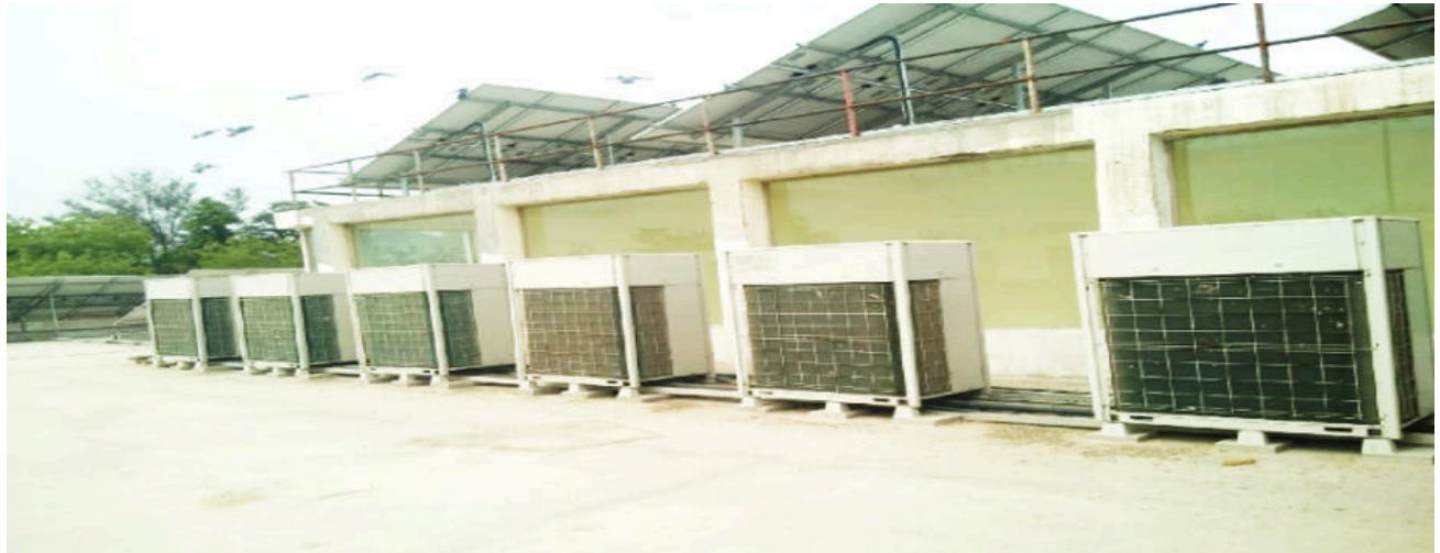
**Figure 3: Variable Refrigerant Volume HVAC System**
