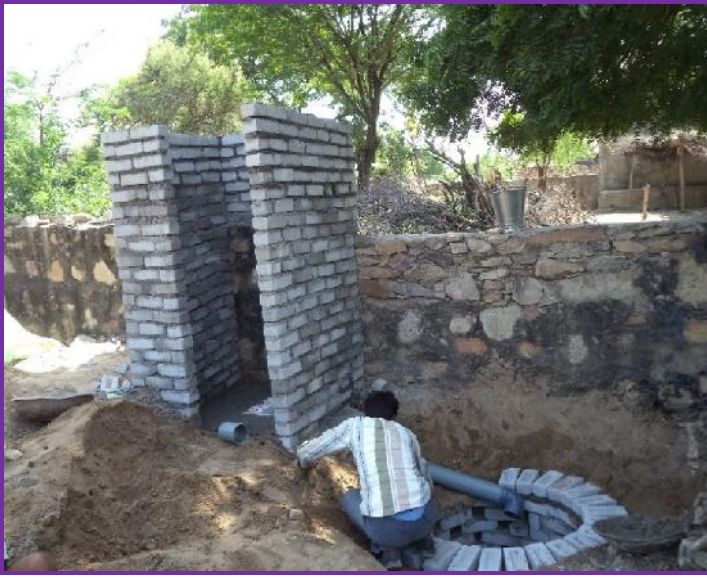
Low Cost Toilet Construction
