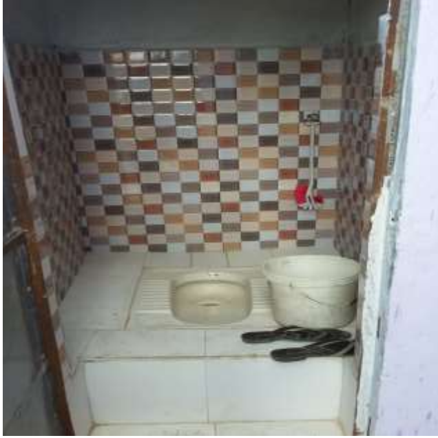
Model toilet constructed at morak
